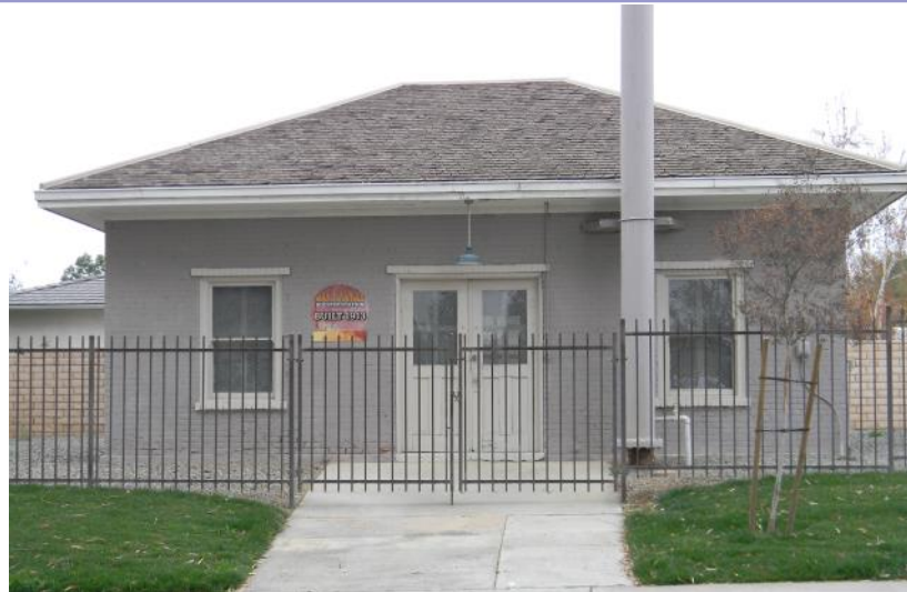
Gage Canal Boosting Station, Built 1913. Mary St.
